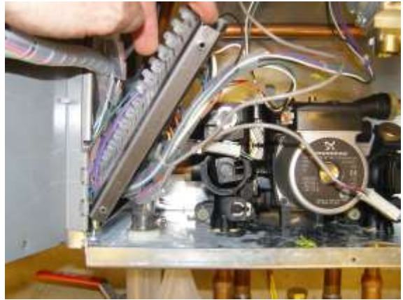
Figure 5: Right retaining clip in locked position
