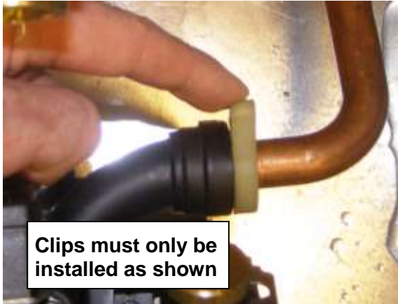
Figure 6: Combi block retaining Clips and Locks
