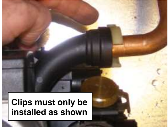
Figure 6: Combi block retaining Clips and Locks
