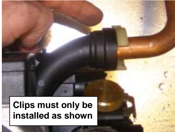
Figure 6: Combi block retaining Clips and Locks
