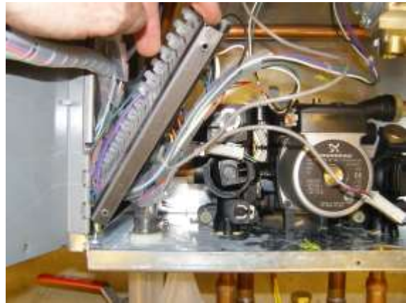
Figure 5: Right retaining clip in unlocked position
