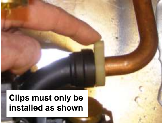
Figure 6: Combi block retaining Clips and Locks
