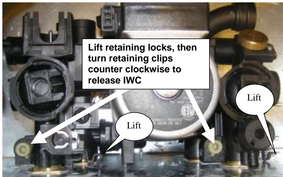
Figure 6: Combi block retaining Clips and Locks
