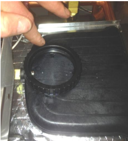
Figure 6 – Installation of New Flue Gasket
