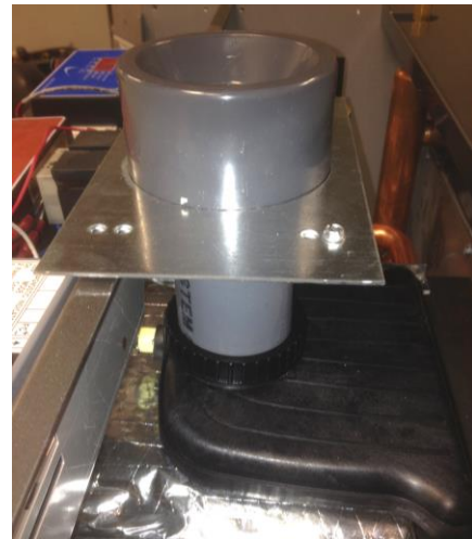
Figure 7 – Installation of New Flue Adapter
