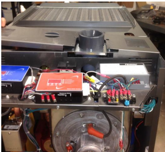
Figure 8 – Reinstallation of Middle Top
